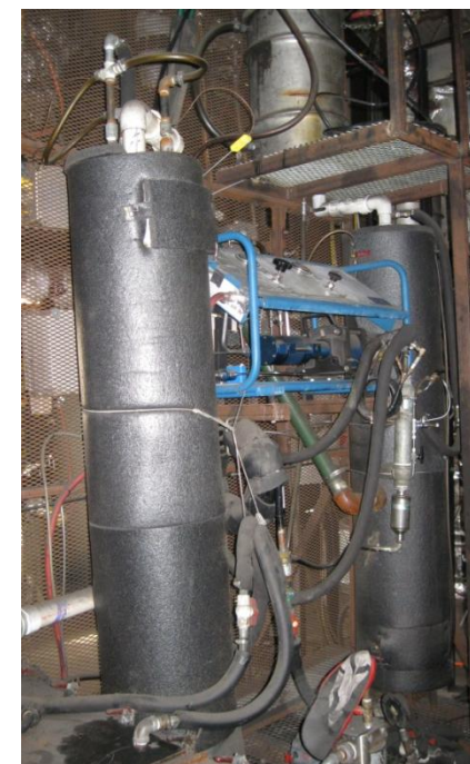
• Gas scrubbing system
