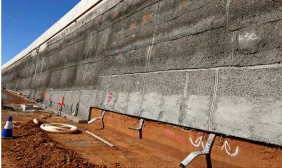
Figure 7. The soil nail wall after full-depth excavation.
