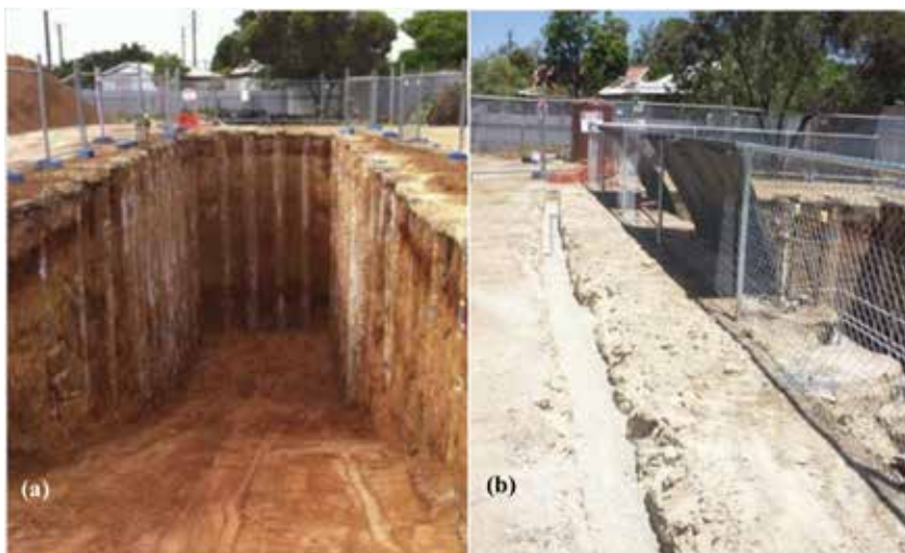
Figure 1. a) A trial pit of up to 8 m in depth, and b) a trench for applying water at the trial.
