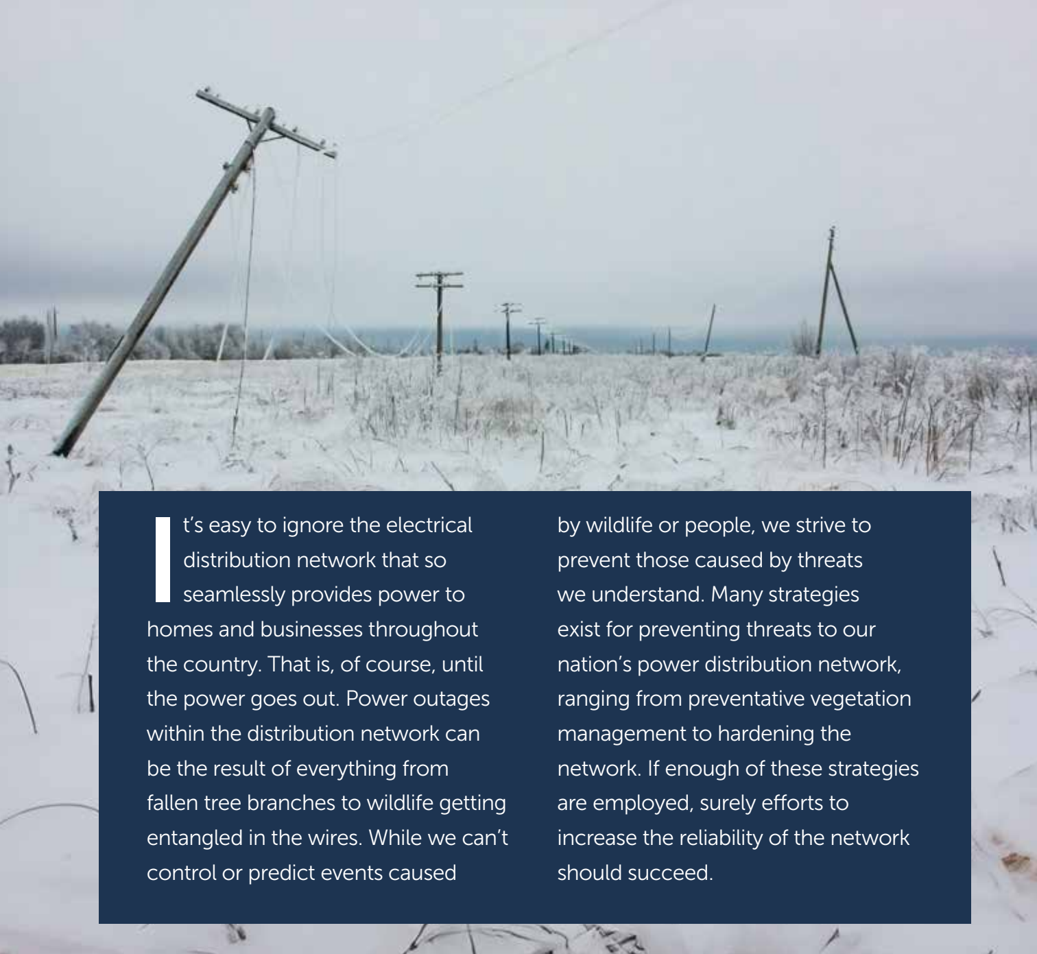
Figure 1. Leaning power poles – foundation failure.
