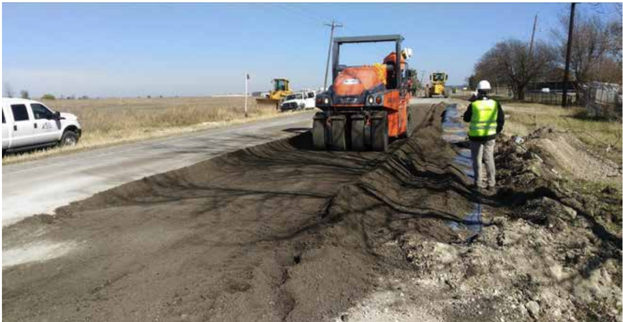
Figure 3. MMG in a reinforced section on FM 1807.
